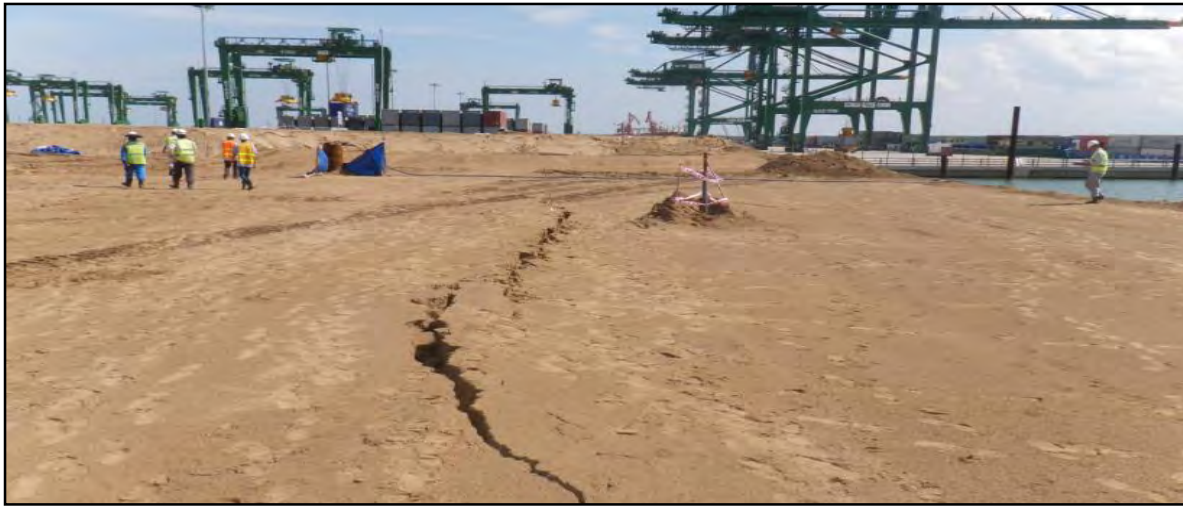
Fig. 1 Downstream view of the first cracks that appeared along the riverbank on April 5, 2010
