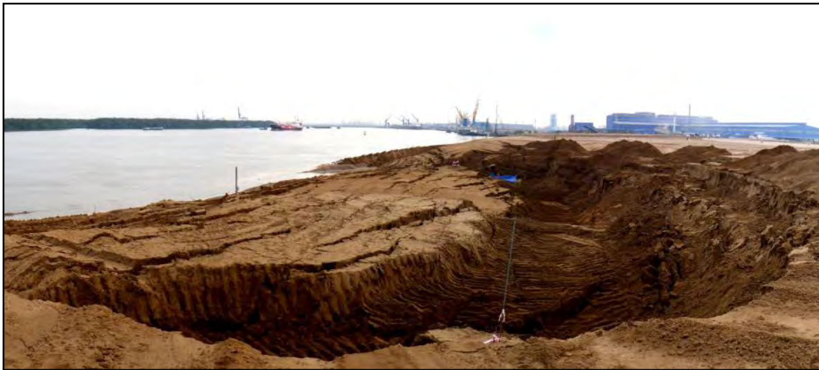
Fig. 2 Slope failure on July 12, 2010, viewed upstream
